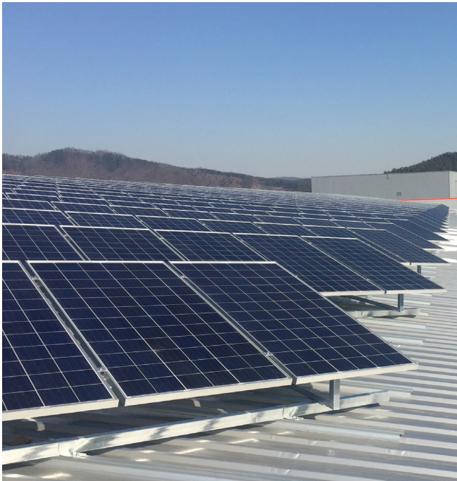
*Dongwon Solar Baekam Industry Solar Power Plant • Location : 859, Baekbong-ri, Baegam-myeon, Cheoin-gu, Yongin-si, Gyeonggi-do, Korea • Generation Capacity : 524.16kW • Shape : Roof attachment type • Completion Date : 2016. 01
